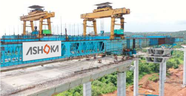
Mopa Airport Link Road
