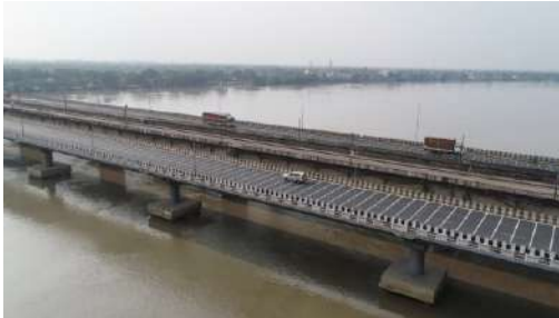
Bridges Across River Roopnarayan
